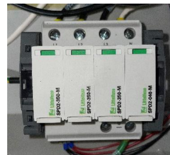
Figure 31 - SPD with four green modules
