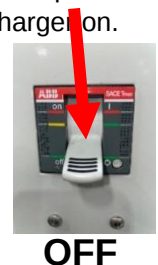
Figure 4—AC main power switch in the OFF position
