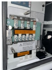
Figure 27—AC main power switch in ON position and LCD display of current power level
