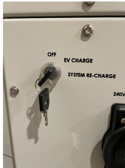
Figure 8—Key Switch in EV CHARGE position
