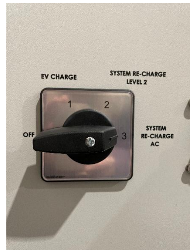
Figure 15—Selector Switch in SYSTEM RE-CHARGE AC (3) position
