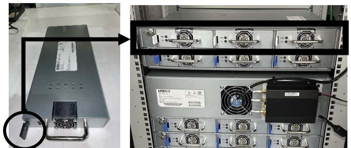
Figure 34 – Inverter modules (white or black tabs) installed in upper shelf of Inverter Shelf Set
